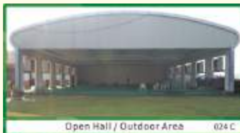
Open Hall / Outdoor Area 024 C
